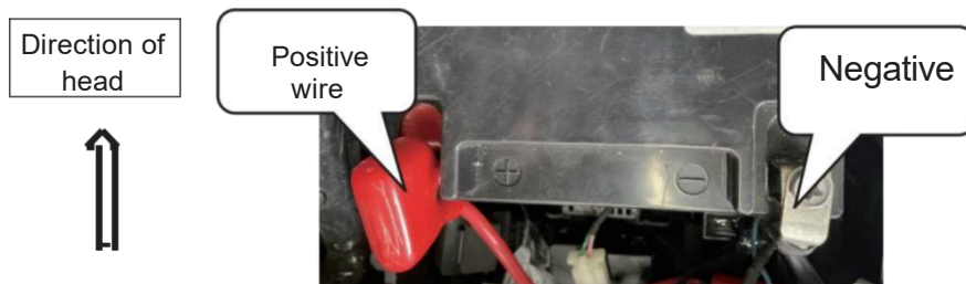
Figure 33 Installation of Battery
